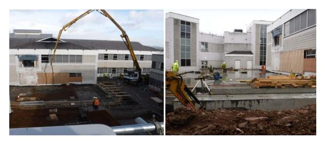
During construction In order to minimise noise disruption and also speed up construction BAM changed the reinforcement from mesh to fibre.
