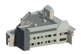
The external envelope comprises a clay facing brick plinth at ground level with composite insulated cladding panels mounted vertically and fixed to steel cladding rails and lined internally with cement bonded particle boards. A proprietary internal shaft wall lining plasterboard system provides 1 hour fire resistance to external walls due to the proximity of the existing surrounding buildings.
